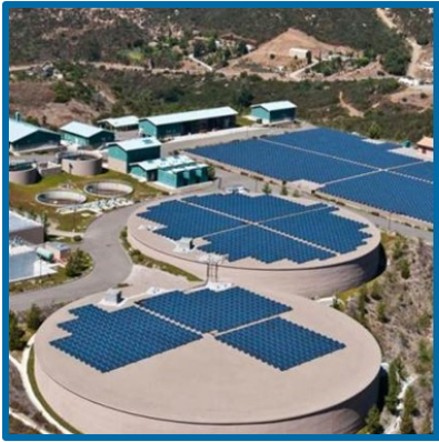
Twin Oaks Valley Water Treatment Plant $179 million
