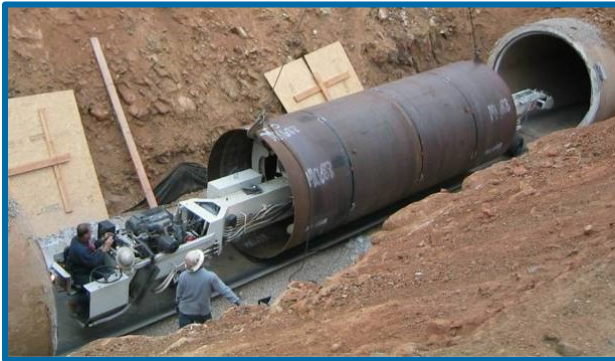
Pipeline Relining $493 million
