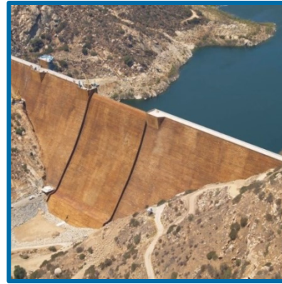
San Vicente Dam Raise & Related Projects $811 million
