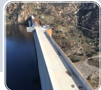
Local Surface Water
