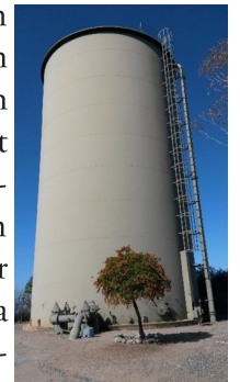
Figure 2 - Abandoned Water Tank to be demolished
