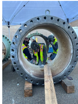
Staff preparing spool pieces for coatings
