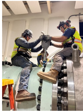
Staff installing air valve on train 4
