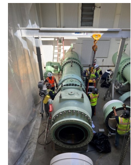
Installation of dresser coupler on high pressure side of train 1
