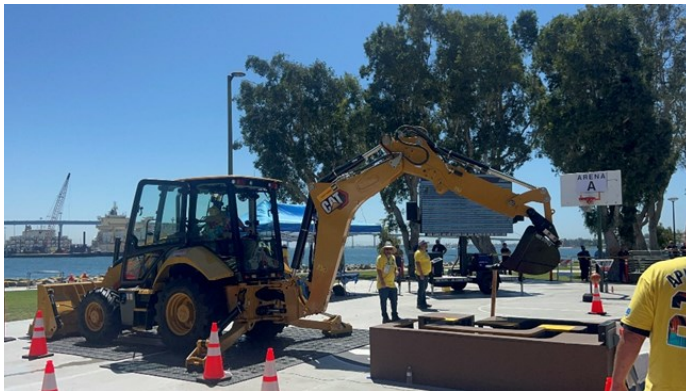
Figure 3 Pictured here are a few of the equipment challenges designed by O&M Facilities Maintenance staff, located in the beautiful Embarcadero
