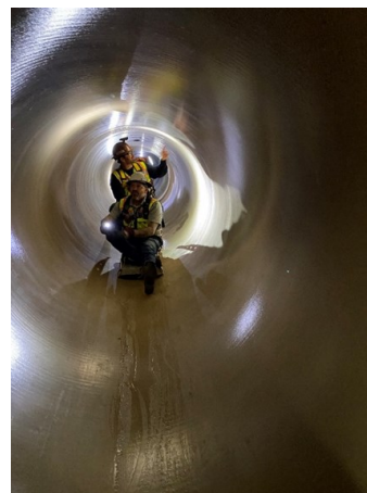
Figure 3: Interior of Fiberglass Reinforced Polymer Pipe
