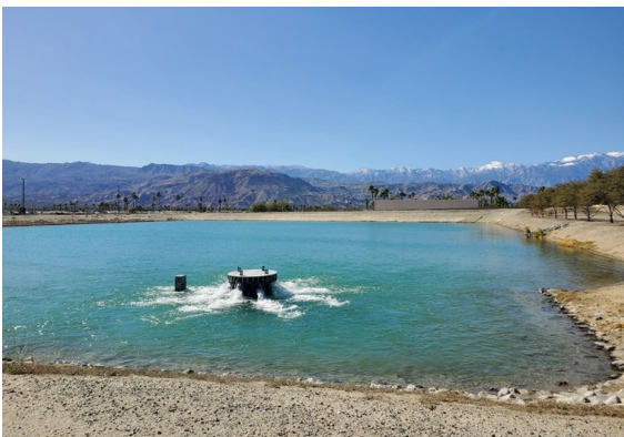
Pictured is a Coachella Valley Water District (CVWD) groundwater replenishment pond, which is sustained by CVWD's Colorado River supplies, and helps maintain that region's critical water aquifer. Photo by Water Resources Specialist Dennis Davis
