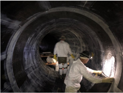
Figure 1: Installation of Carbon Fiber Reinforced Polymer Liners
