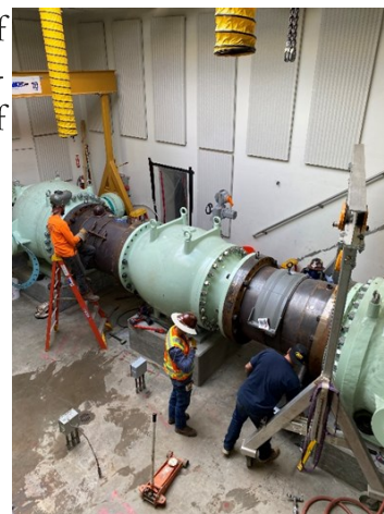
Figure 3 - New Valve and Pipe Installation
