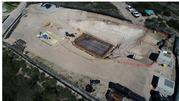
Drone photos of Flow Control Facility work site taken February 26, 2021
