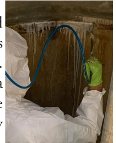
O&M Crews Injecting Foam Product
