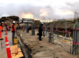
Figure 3: Electrical Building Conduit Preparation
