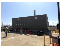
Figure 4: Electrical Building completion
