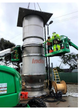
Figure 1: Pump Installation (shipped from Spain)
