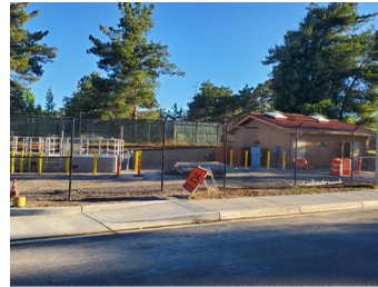
Vallecitos Water District 11/Vista Irrigation District 12 Flow Control Facility (newly constructed facility)
