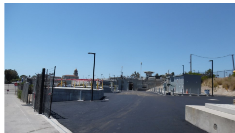
San Diego 28 Flow Control Facility – Exterior of New Facility
