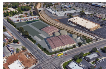
Escondido Membrane Filtration Reverse Osmosis Facility
