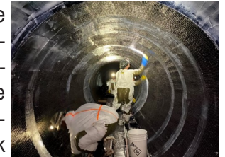
Figure 3 - Carbon Fiber Liner Installation
