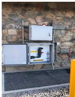
Figure 2 Chemical Fill Station
