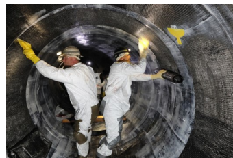
Pipeline 4 Carbon Fiber Liner Installation
