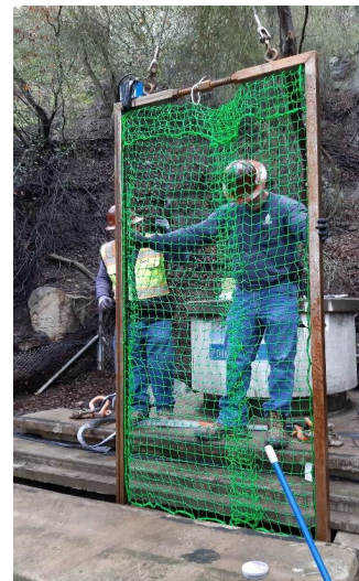
In-house designed and fabricated catch net. The frame can be adjusted to accommodate varying channel widths
