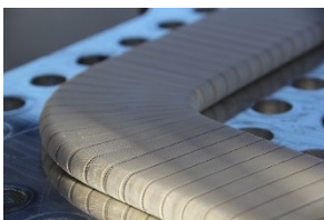
Close-up view of newly insulated and cured bus bar
