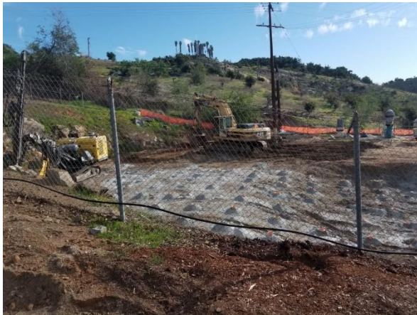
Holes drilled to insert blasting charges.
