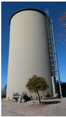
Figure 2 Abandoned Water Tank
