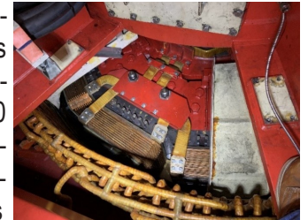
View of a set of bus bars, clamping plates and rim studs
