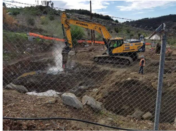
Attempts to remove granite prior to blasting.
