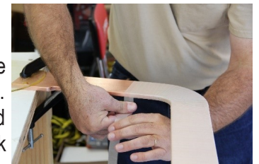
First of five different tapes being applied on a bus bar
