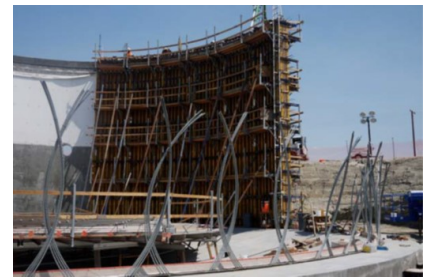
Figure 3 Prestressed Concrete Reservoir
